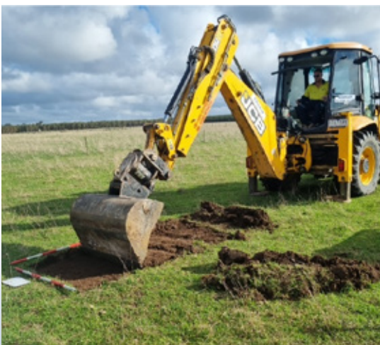
Above: Digging a test pit to learn more about the local soil conditions Below: We completed ground investigations along the transmission route this year
