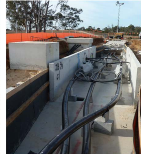
Joint bay construction
