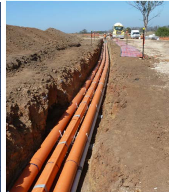
Conduits in trench (cables go inside)
